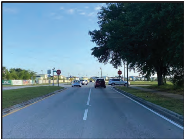
Looking north towards the intersection
