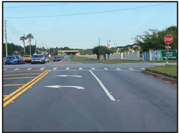
Looking west towards the intersection
