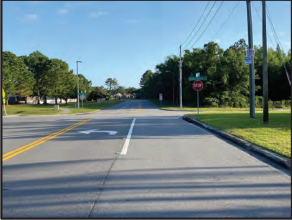
Looking north towards the intersection
