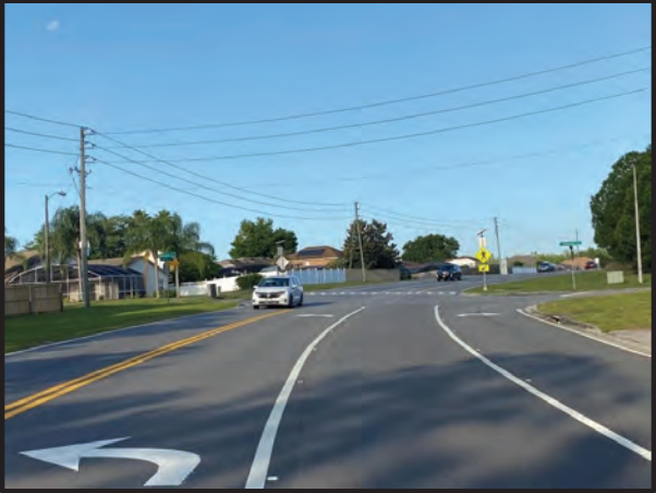
Looking west towards the intersection
