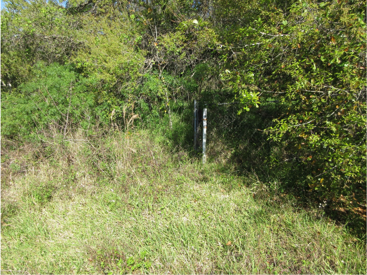
Buried Fiber on Upstream side
