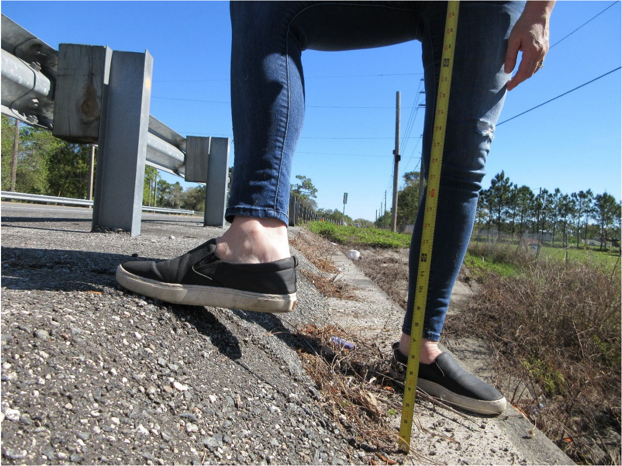
Asphalt at Headwalls
