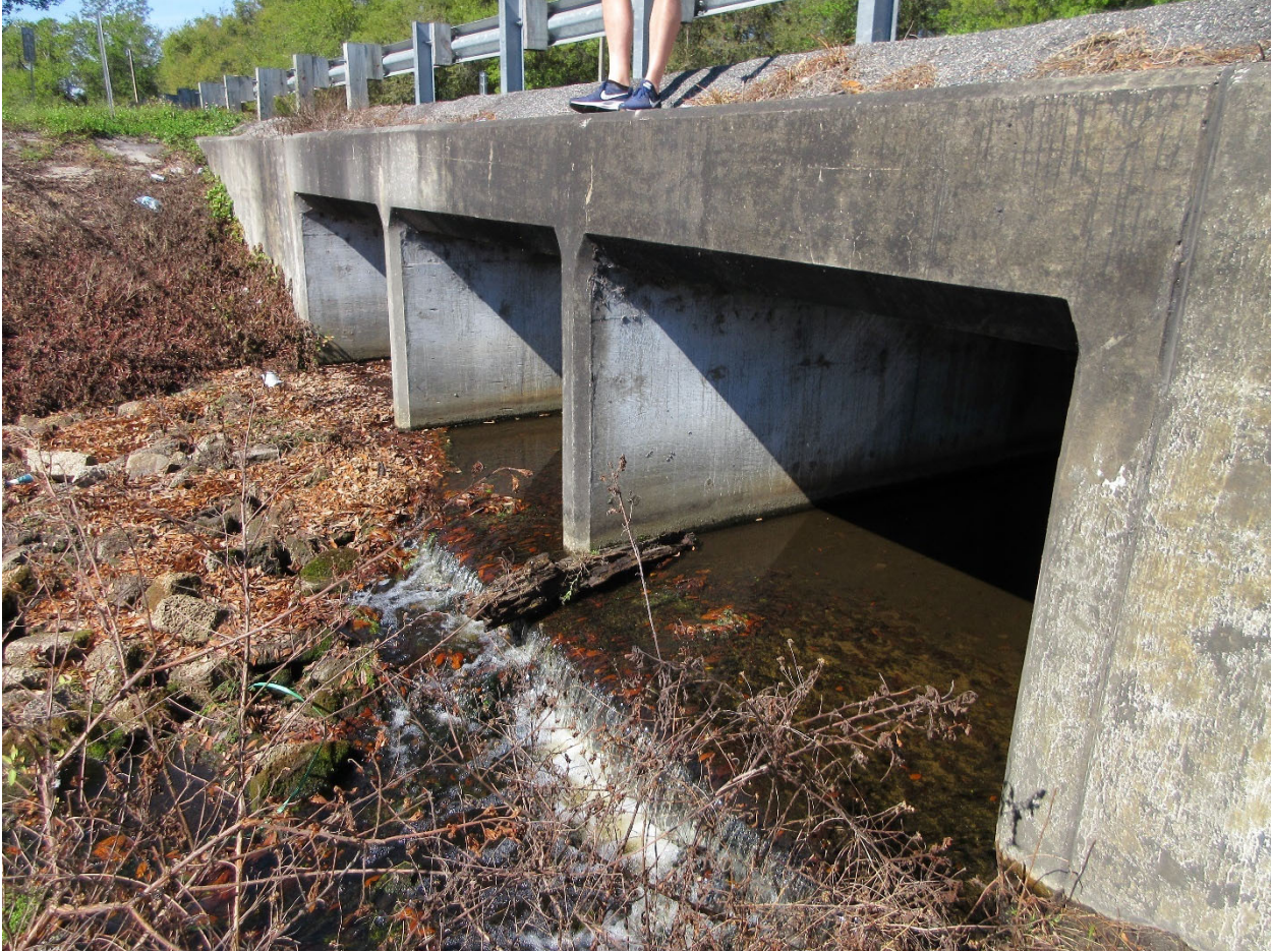
Cutoff Wall Exposed
