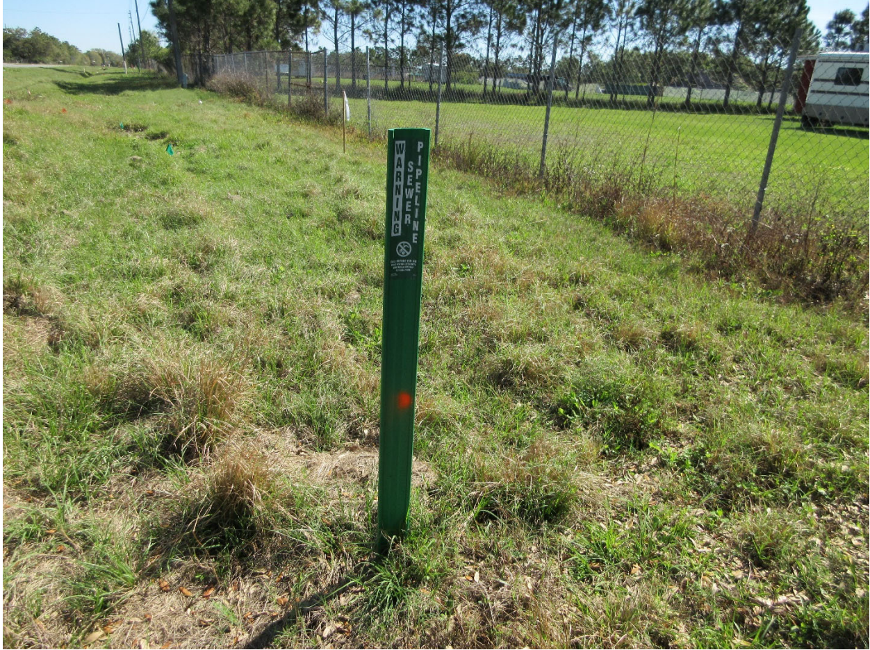
Sewer Utility on downstream side
