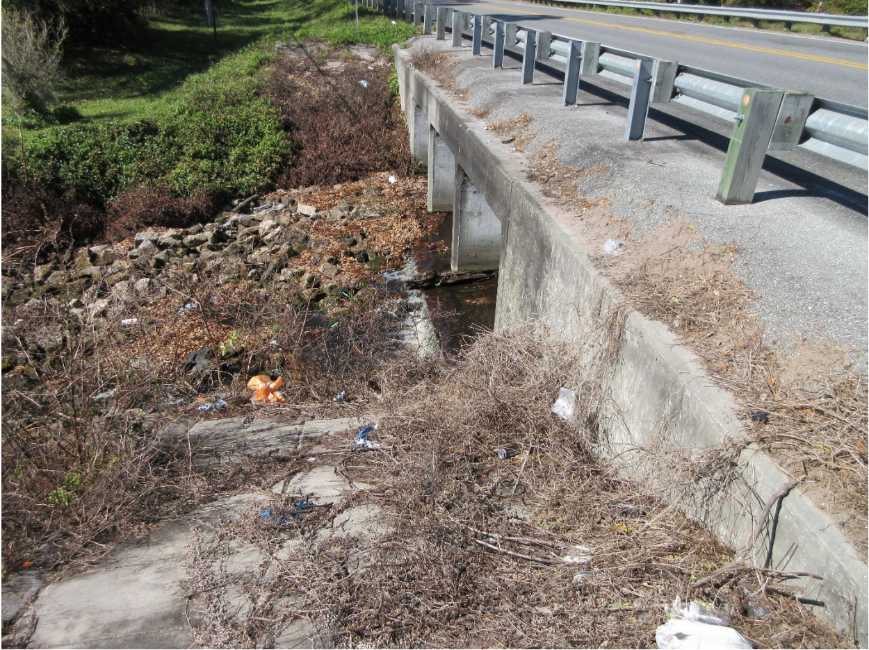
Culvert Opening Downstream
