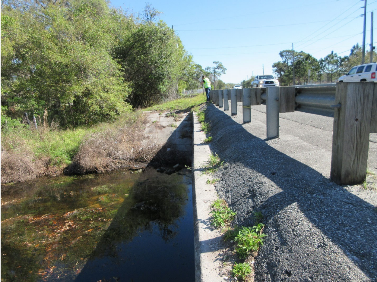
Culvert Headwall Upstream
