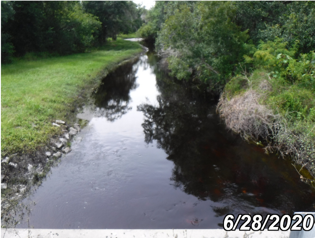
Channel Looking North
