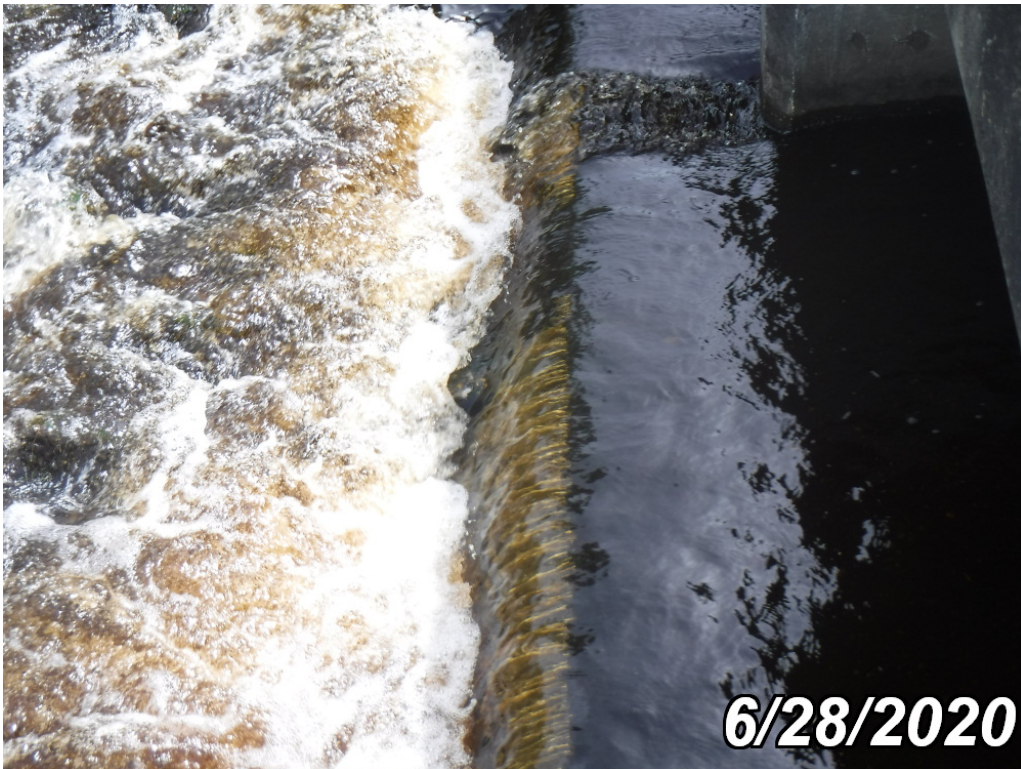
Photo 2: Element 8290: South toe wall exposure at Cell 3.
