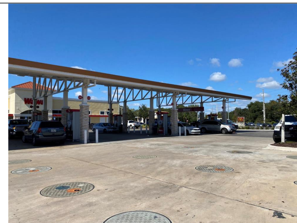
View across the facility from the southeast corner facing northwest, towards the dispensers and convenience store.
