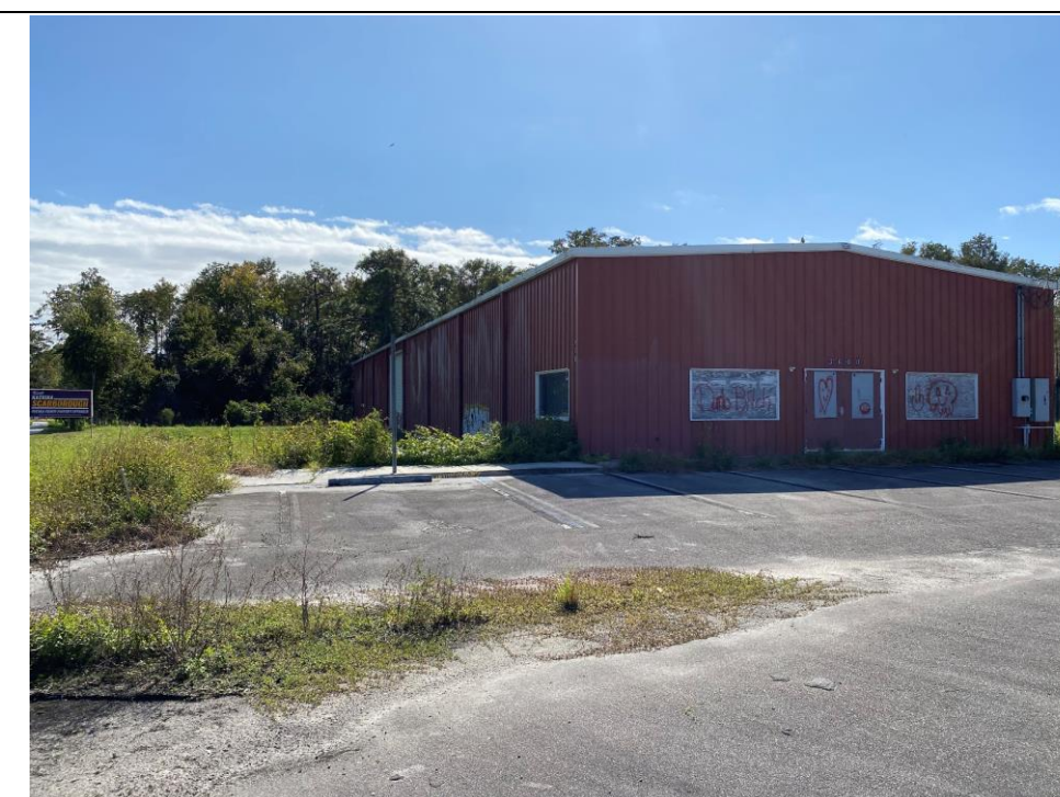
View of the vacant warehouse and paved parking area on the northern side of the property.
