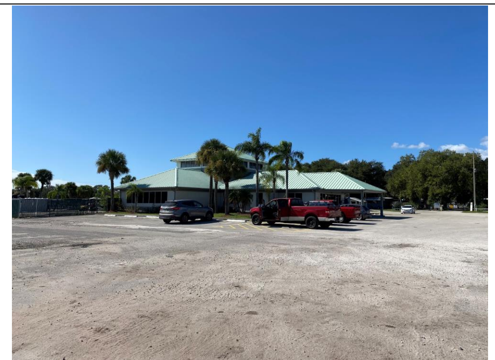
View of the office building at the north end of the property, facing southwest.
