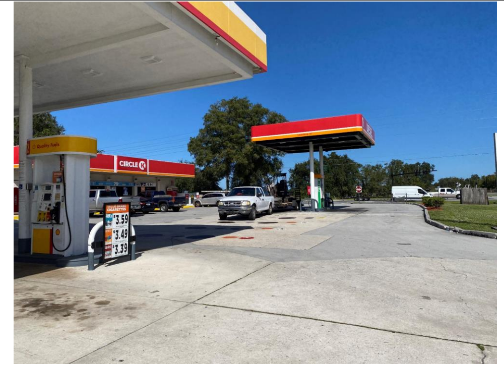
View of the gasoline dispenser island (yellow canopy), convenience store (far left), UST field (center), and diesel dispenser islands (red canopy) from the southeast corner of the site, facing northwest.
